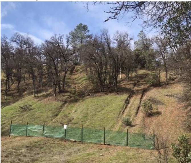
One of five fence barriers installed in February
