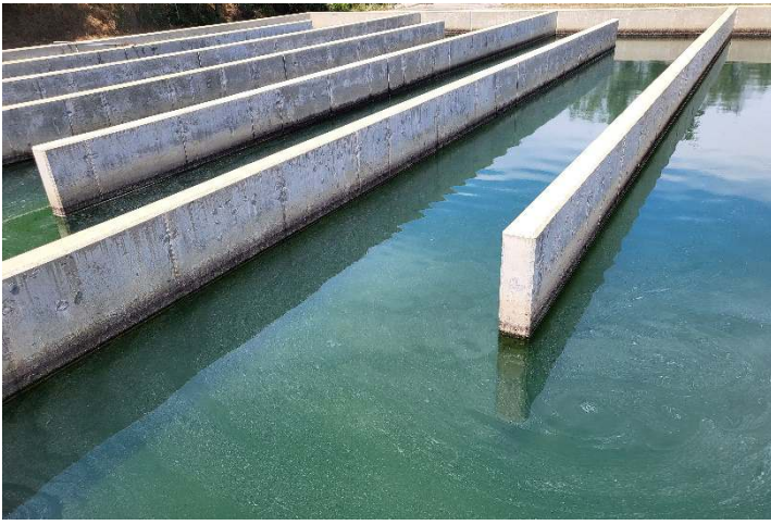
Treated water ready for filtration and chlorination steps.
